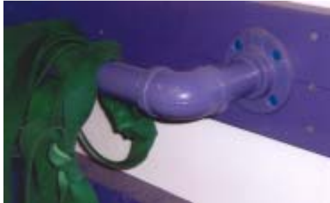
^Lower level of pipes (bottom three rows are hooked the same.)
