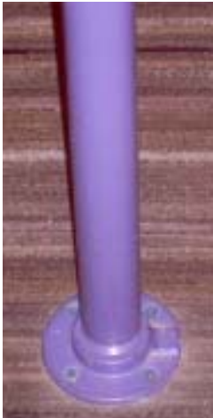
^Pipes bolted into the floor
