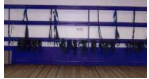
Right Side Wall Pipes
